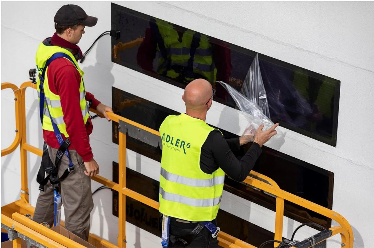
Caption 3: With the help of the integrated adhesive on the back, the HeliaSol<sup>®</sup> solar films can be precisely attached by the assembly team.
