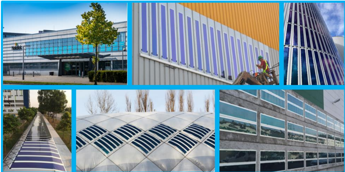
Figure 3 – Pilot installations from all over the world
