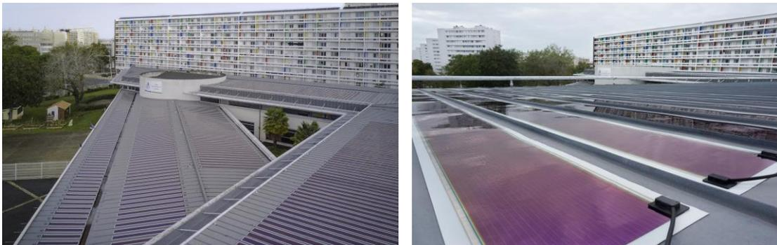
BiOPV roof installation in La Rochelle, HeliaSol<sup>®</sup> on standing seam roof system - © Heliatek GmbH
