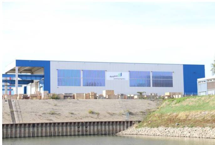
Organic photovoltaic facade - port of Duisburg, © duisport
